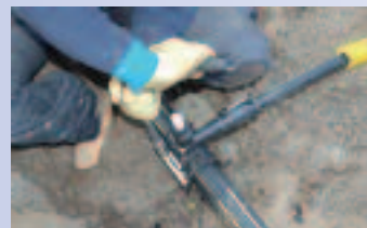
Pose de raccord
